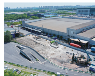
Construction on ZF's expansion project is in full swing. — Zhang Jian
