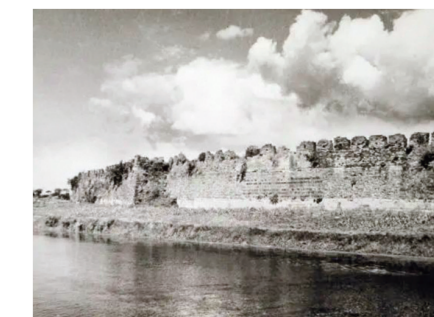
In the spring of 1951, only the northern side of the West Wall remained standing.
