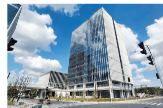
The first phase of the project includes the completion of 14 buildings. — Zhang Jian
