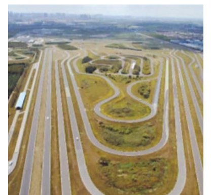
The Anting Test Track features various road surfaces for different testing purposes. — Hu Xindong
