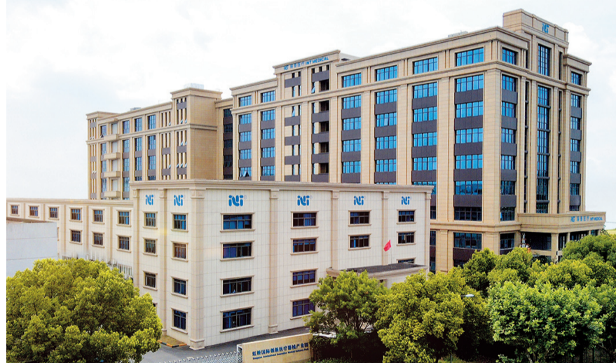
The Hongqiao International Innovative Medical Industrial Park in Jiangqiao Town — Li Huacheng
